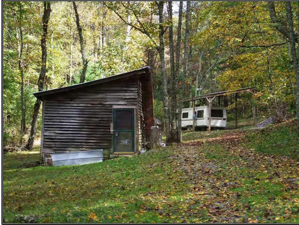
Figure 19. View of the hunting cabin on the east side of Martin Gambill Road, facing east.
