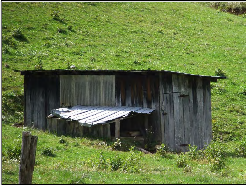
Figure 14. View of the second shed, facing west-northwest.
