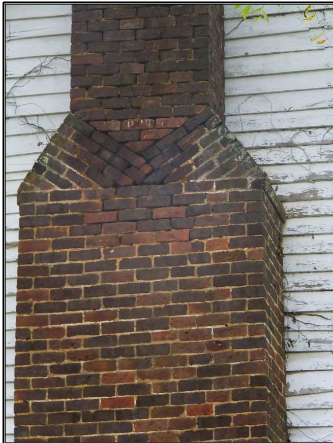
Figure 33. Detail of the brick chimney on the northeast elevation, facing southwest.
