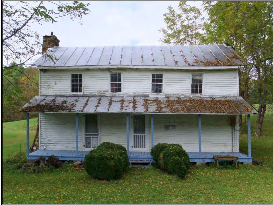
Figure 30. View of the façade of the Stephen Ward House, facing north-northwest.
