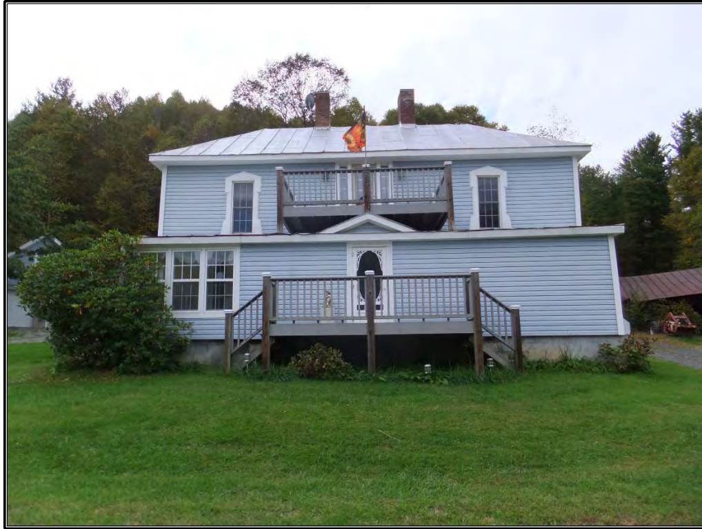
Figure 51. View of the façade of the Frank Edwards House (circa 1900), facing west.
