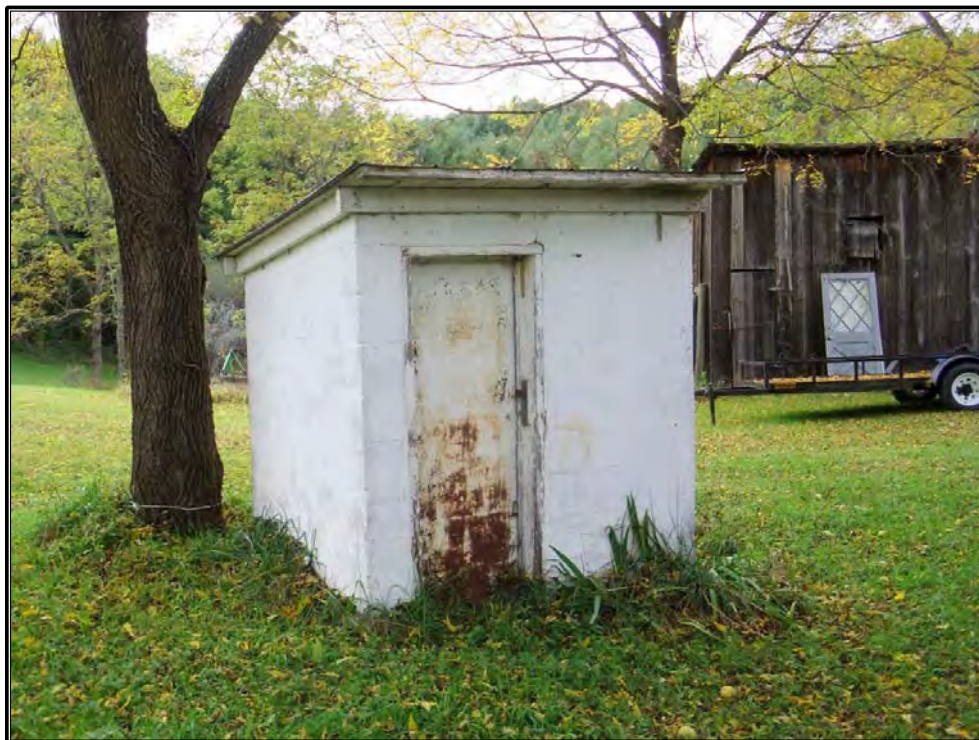
Figure 36. View of the circa 1900–1956 pump house, facing west-southwest.
