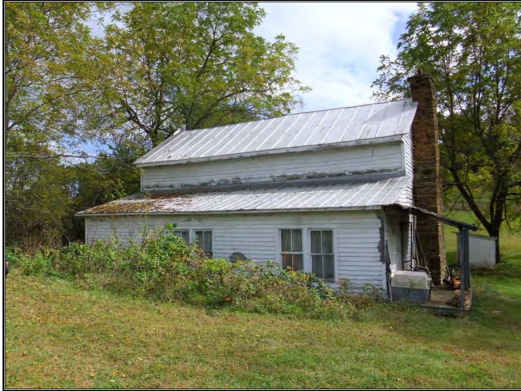
Figure 34. Detail of the rear, or northwest, elevation, facing south-southeast.
