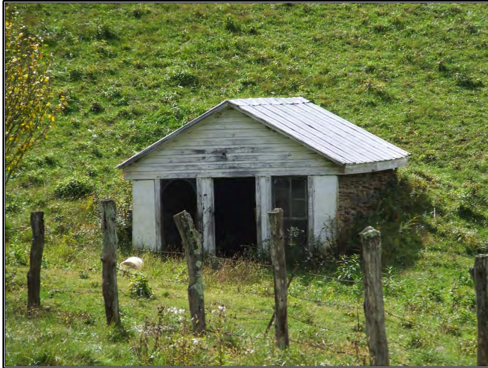
Figure 15. View of the cellar/canning house, facing west.
