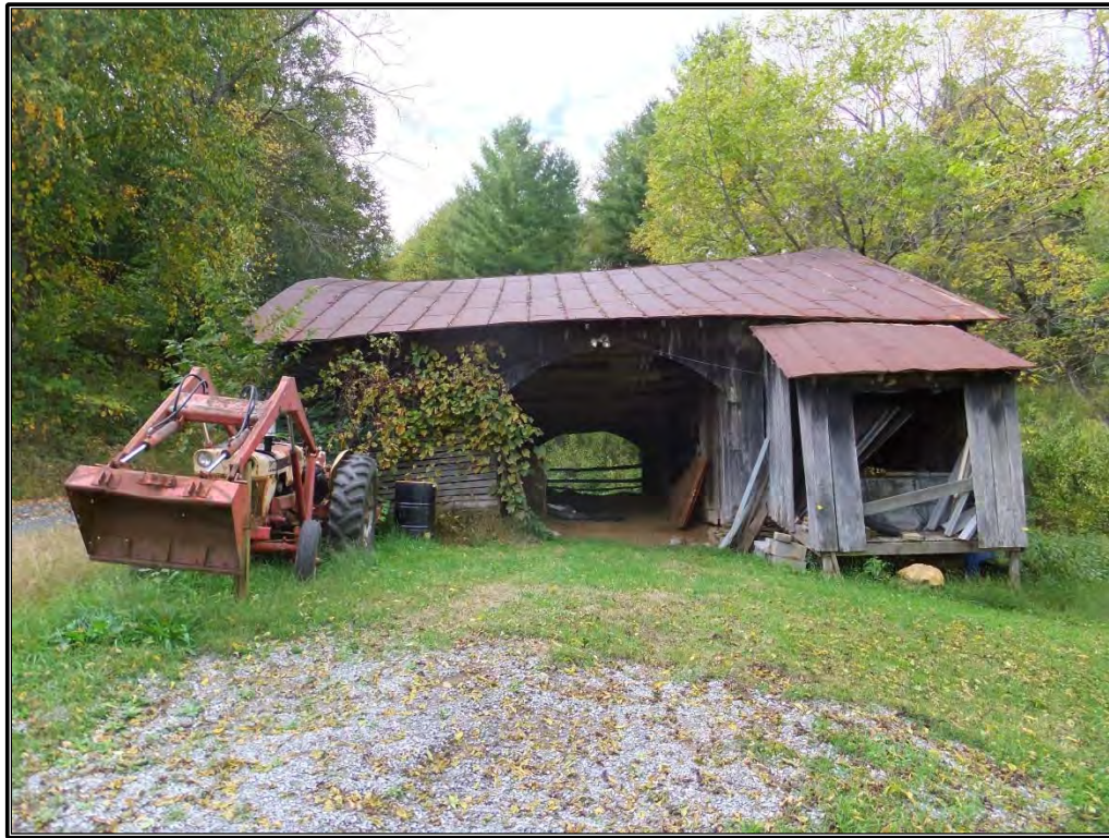
Figure 57. View of the east elevation of the barn, facing northwest.
