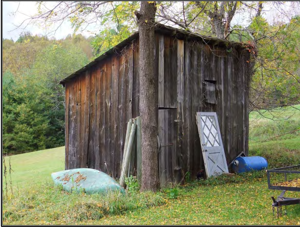
Figure 37. View of the circa 1950–1970 shed, facing northwest.
