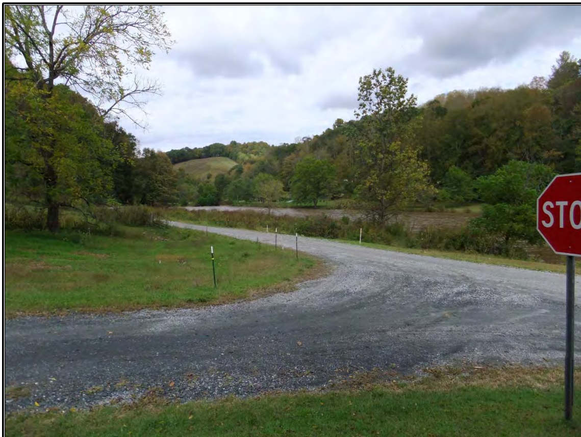
Figure 46. View of the intersection of Martin Gambill Road and Garvey Bridge Road to the east of the South Fork New River, facing north.
