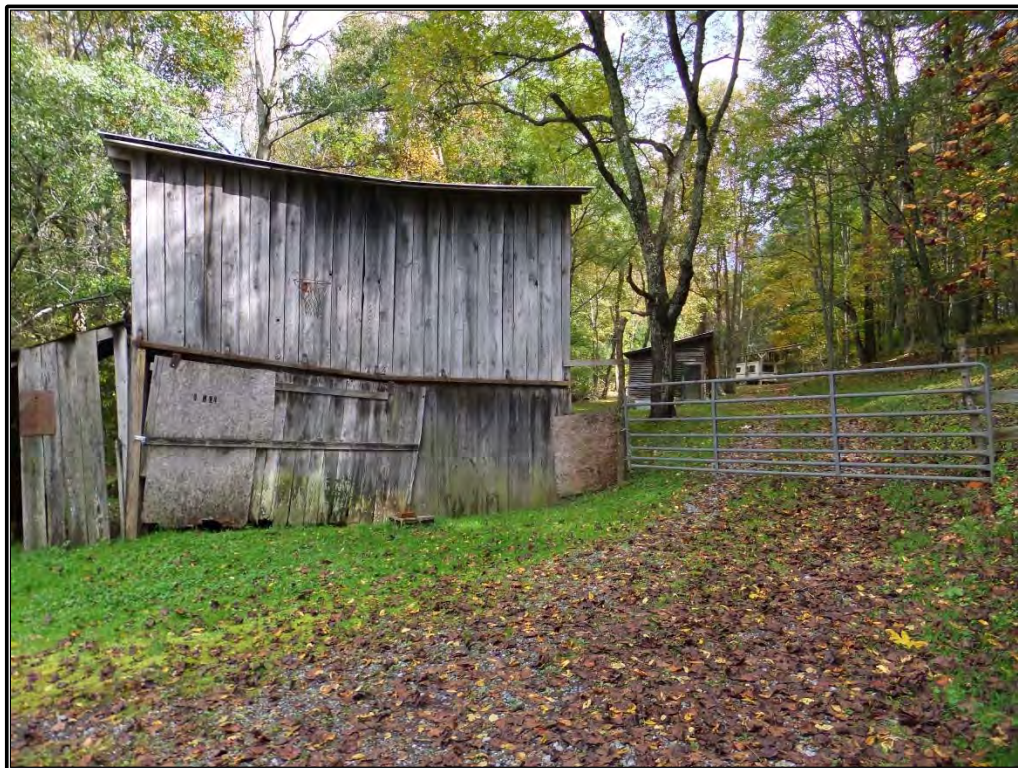
Figure 6. View of the barn, hunting cabin, and modern carport associated with the Ward Farm (AH0202), facing east.
